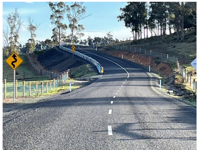
Safety has been improved through new advisory signage, line marking, guidepost and roadside barrier. Photo source: Dorset Council
