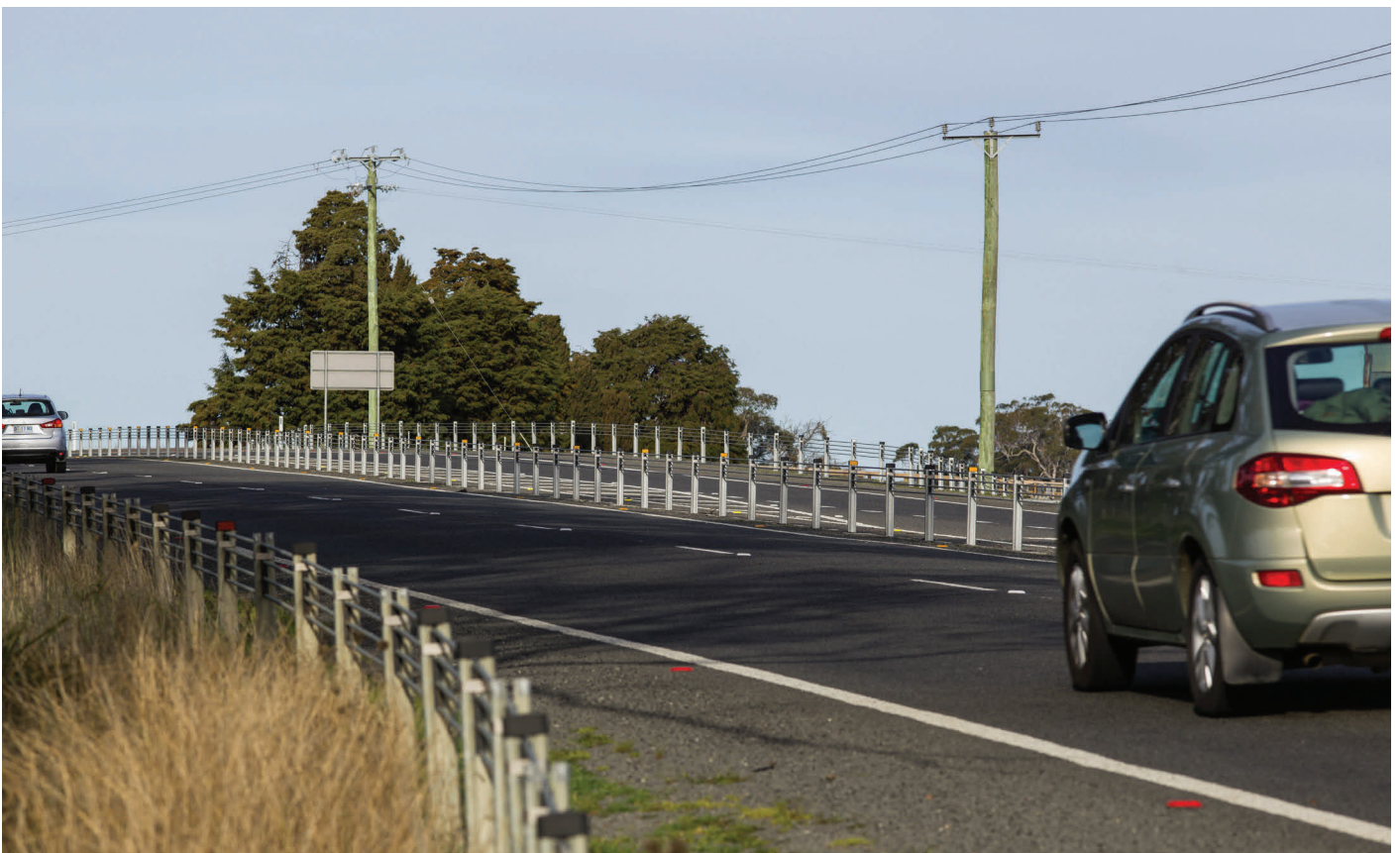
Flexible safety barriers provide full separation between vehicles travelling in opposing directions.
