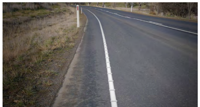
Sealed shoulder provided with audio tactile edge line
